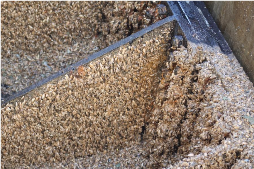
Figure 7. Eight years' worth of quagga mussels accumulated on a wheel gate pulled out of the water for maintenance at Glen Canyon Dam, Arizona. These nonnative species anchor themselves to nearly any surface near running water and reproduce rapidly. Mussel populations have covered boats, marina docks, motors, pipes and other water works in many Reclamation infrastructures, reducing the efficiency of these resources.
