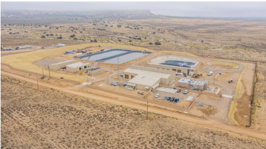
Figure 10. Navajo-Gallup Water Supply Project - Aerial image of the Cutter Lateral Water
