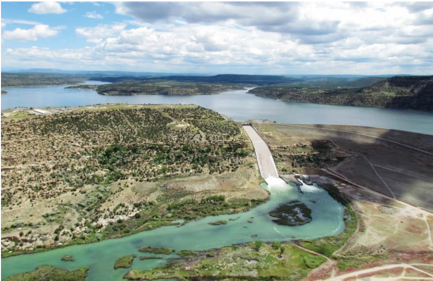
Figure 5. Water from Navajo Reservoir is released down the Navajo Dam spillway. The dam is located on the San Juan River, 34 miles east of Farmington, New Mexico. (Reclamation photo by S. Pernick)
