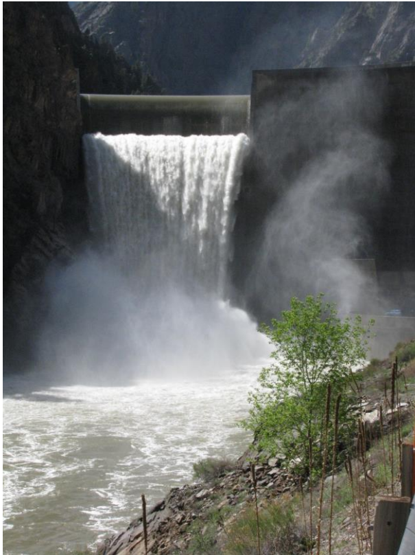
Figure 6. Spillway at Crystal Dam located six miles downstream from Morrow Point Dam and 20 miles east of Montrose, Colorado. This hydropower dam is part of the Aspinall Unit, a set of three dams on the Gunnison River that are all part of the Colorado River Storage Project.
