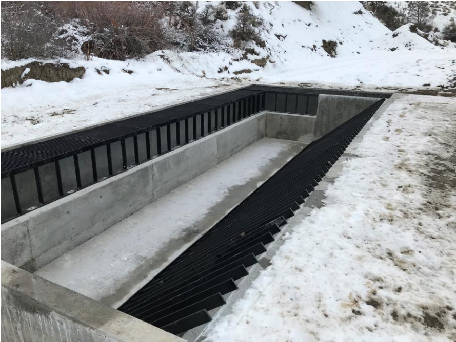
Figure 13. Intake structure for Upper Stewart Ditch Project in Paonia, Colorado.
