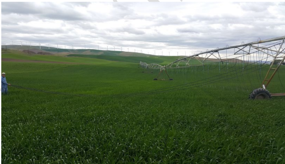
Figure 61. MDI installed on a center pivot while retaining the sprinklers for switching between MDI and MESA. The driplines on the outside spans of the pivot are longer since it covers a larger area in the field. Although the crop is wheat, the MDI system is set up for taller crops.
