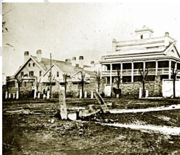
Figure 3. Irrigation ditch outside Brigham Young's Beehive and Lion houses ("Using Water: Irrigation")
