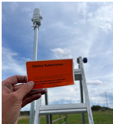
Figure 3. Atmos 41W weather station installed with subscription details.
