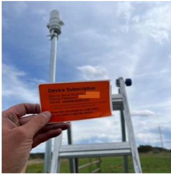
Figure 11. ATMOS 41W weather station installed
